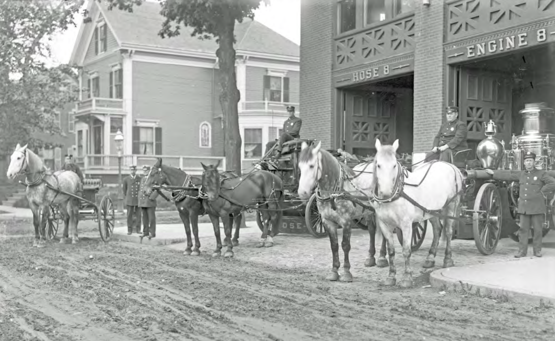
536 Deering Avenue Engine Co. No. 8 Firehouse, 1907
