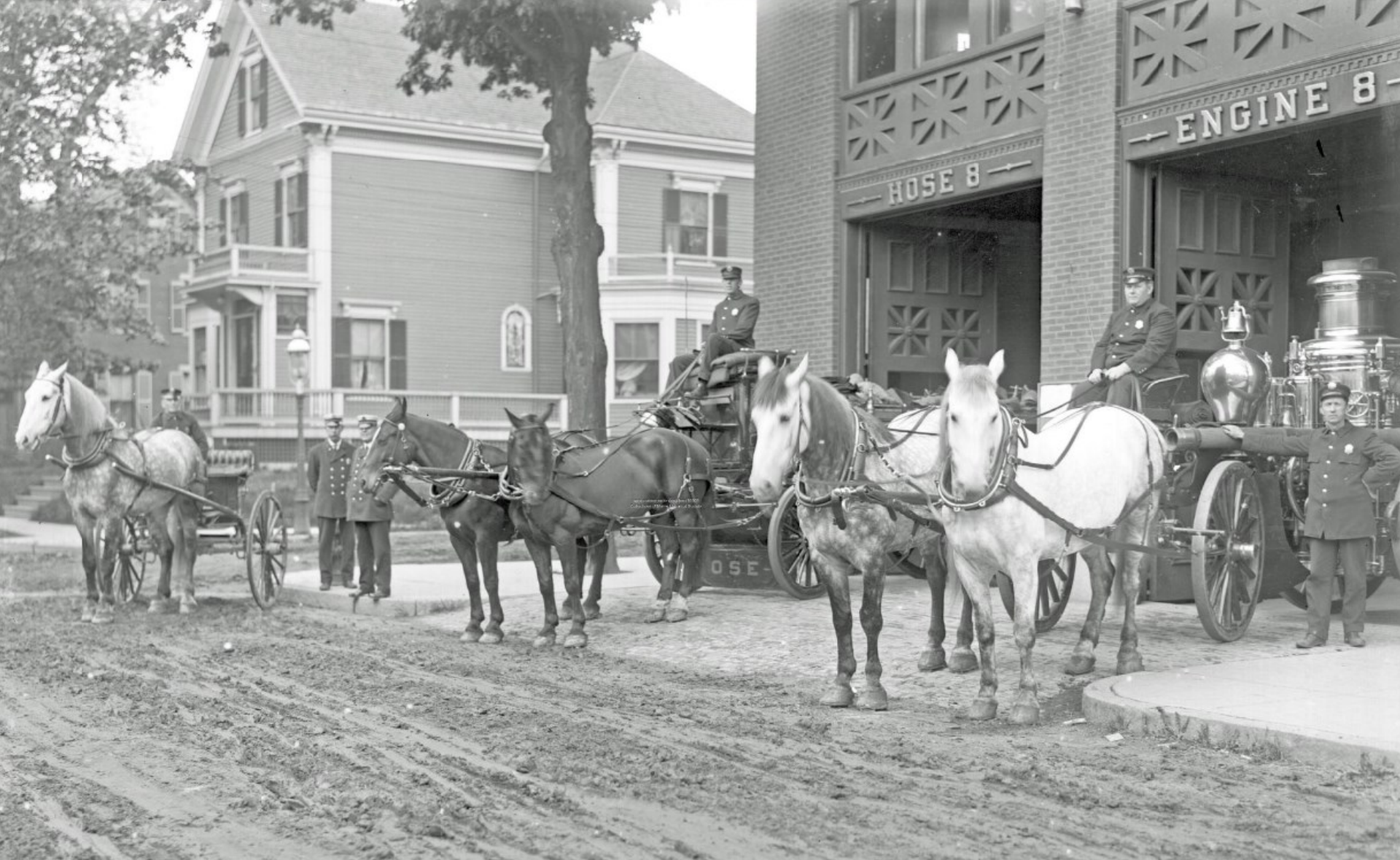
536 Deering Avenue Engine Co. No. 8 Firehouse, 1907
