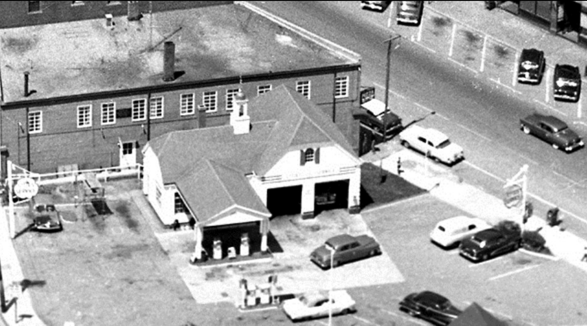
634 Forest Avenue Jordan Automobile Service & Filling Station, 1934
