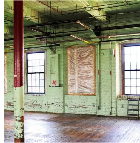
Bates Mill No. 2 BEFORE redevelopment
