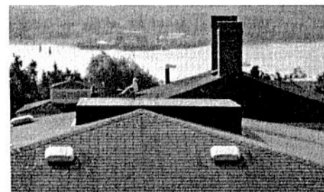
With modern heating systems, the common chimney will increasingly become an endangered building element.
