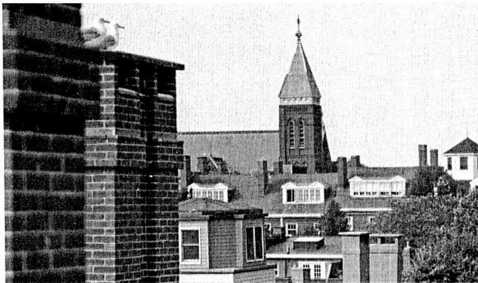
GPL restored the Safford House chimneys (left) to last another 100 years.
