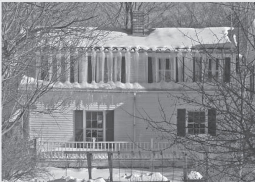
Improperly installed weatherization retrofits can do more harm than good. Above, heat tape simply transfers an ice dam problem from the roof to the space below. Below left: Squirrels entered the gaps in this attic and disrupted the insulation.
